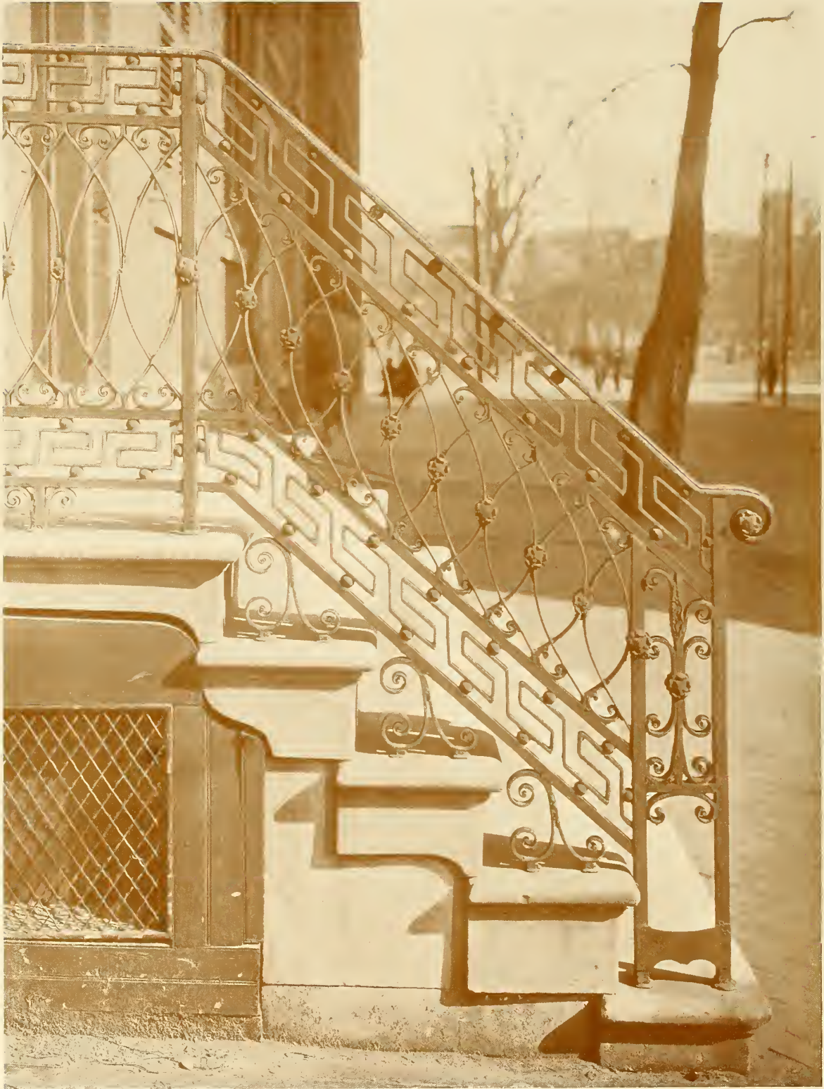
BALUSTRADE, NO. 711 LOCUST STREET Philadelphia
